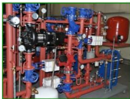
Thermal Heat Distribution
