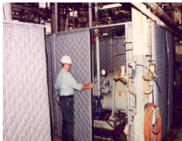
Typical double track design sliding panel access for compressor enclosure.
