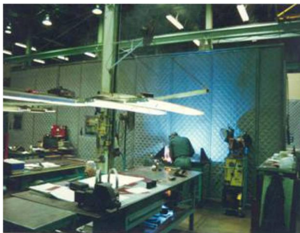
ABAC high temperature 12' high curtains protect a welder from brake and shear noise in a machine shop.
